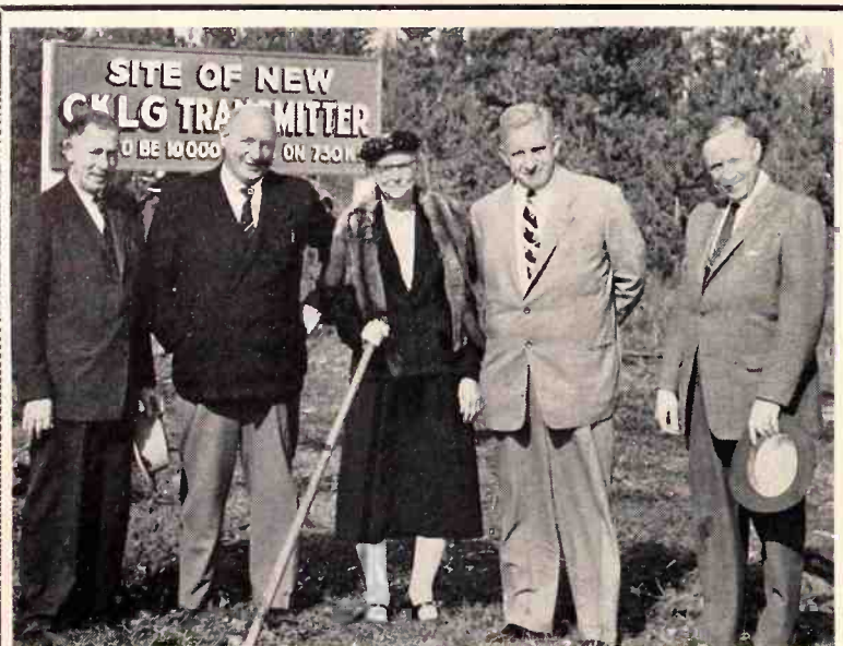
First sod was turned at new CKLG transmitter site near Ladner by 86-year-old Mrs. W. F. Gibson. She is seen flanked by her four sons: Jack, Clark, Gordon and Earson Gibson, owners and operators of CKLG.
