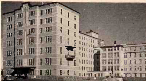
Rimouski's new modern hospital.
