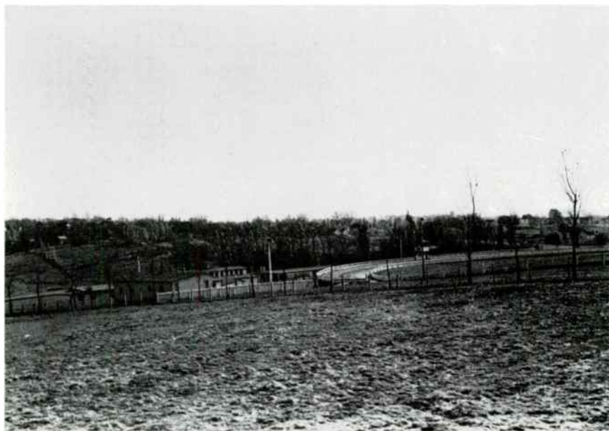
Site of proposed tower at Silver Acres (Pennsylvania Avenue) looking Southeast—1938
