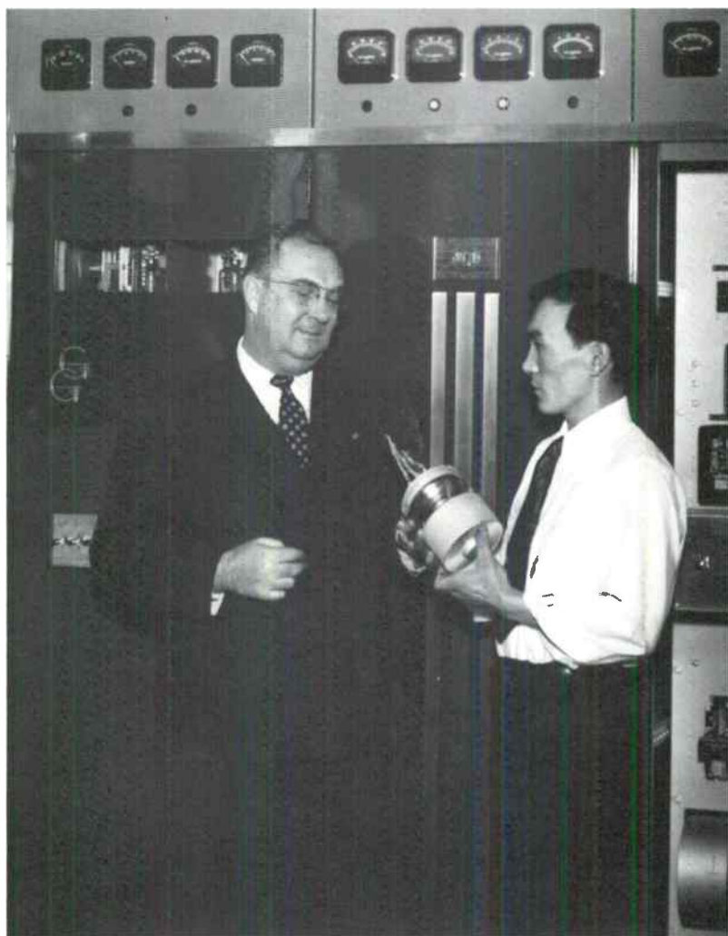
New RCA transmitter at WDBQ (Jim Carpenter and John Uyeoka)
