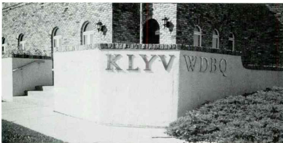
Broadcast Center at 5490 Saratoga Road in Asbury, 1987-
