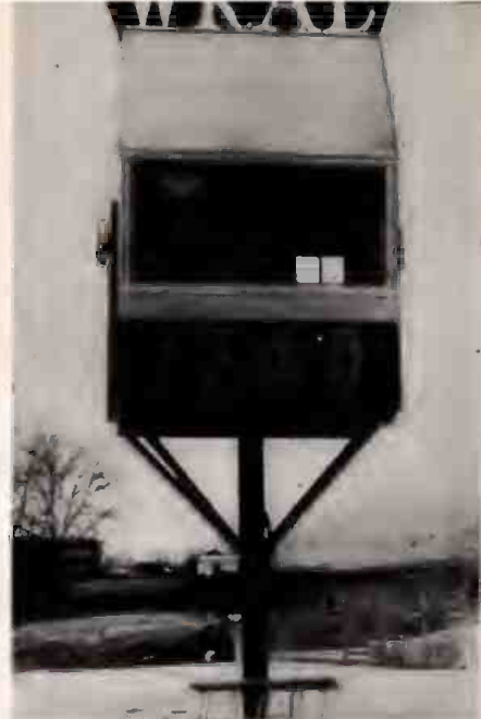
This is the house that WRAL built on U.S. Highway 1 from which it broadcasts to a traveling audience. Building rotates north and south to face morning, evening traffic.
