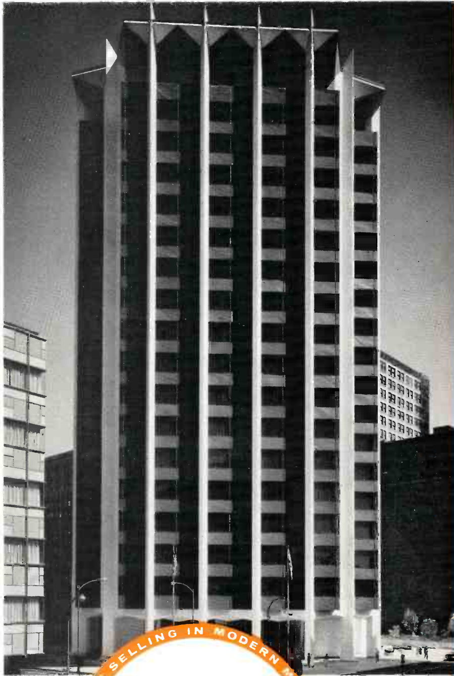
THE MULTI-AWARD WINNING UNITED STATES GYPSUM BUILDING, CHICAGO
