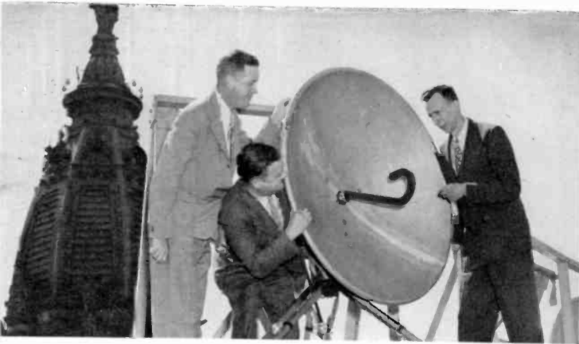
Above: WBZ-TV's chief engineer W. H. Hauser (right), George E. Hagerty (left) engineering manager of Westinghouse Radio Stations, Inc., and J. K. Hiller of RCA check the microwave equipment for the Boston station, due to open late this year.
