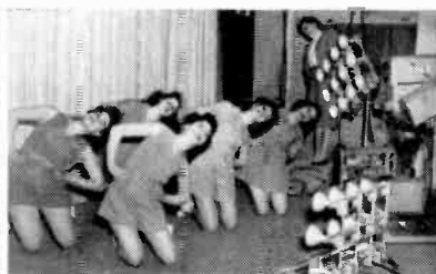
★ Station WBKB, Chicago
