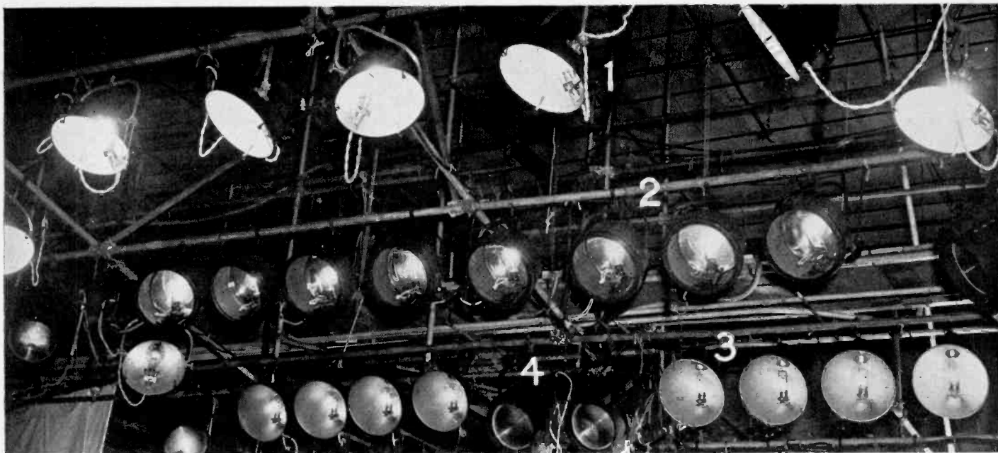
Lights Used at WCBW-CBS: 1 & 2) Century Projection Spots, 3) Kliegl Elliptical Floods, 4) Century 5000-Watt Spots. Salzman and Duarcs Not Shown.
