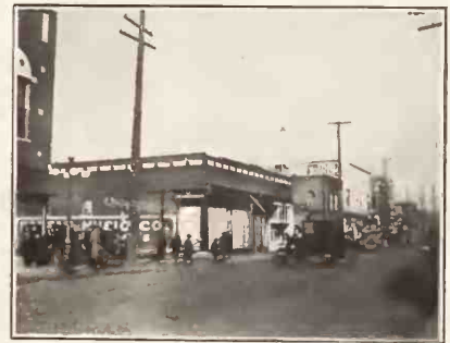
Morgan Co. in Tornado Belt
