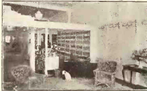
A corner of the new Victor department of Griswold, Richmond & Glock, Meriden, Conn., considered one of the finest retail talking machine warerooms in New England.
