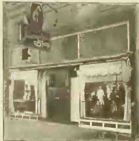
Exterior of Peerless Phono. Shop
