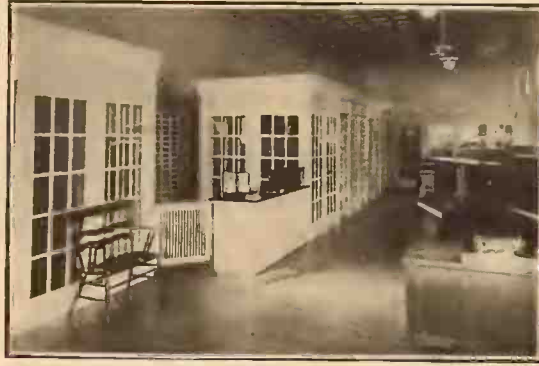
General View of Interior of Store
