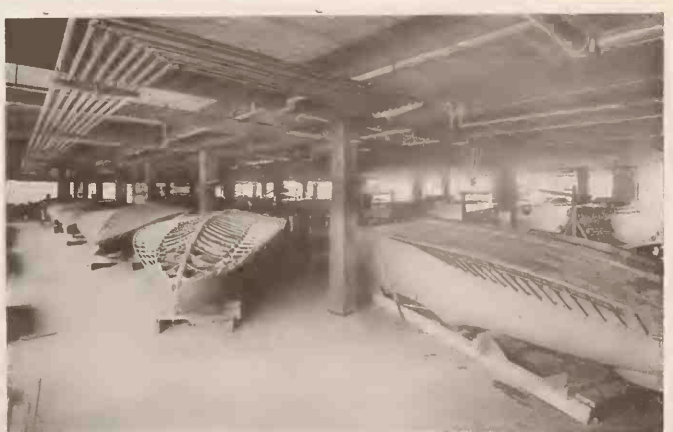
Hydro-Planes in Course of Construction at Unico Plant
