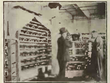
Shows Stock of Heineman Motors
