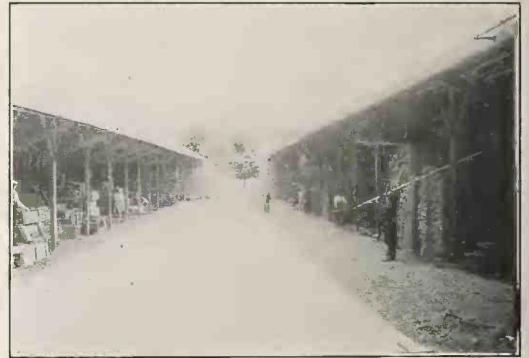
Covered Veneer and Lumber Sheds.
