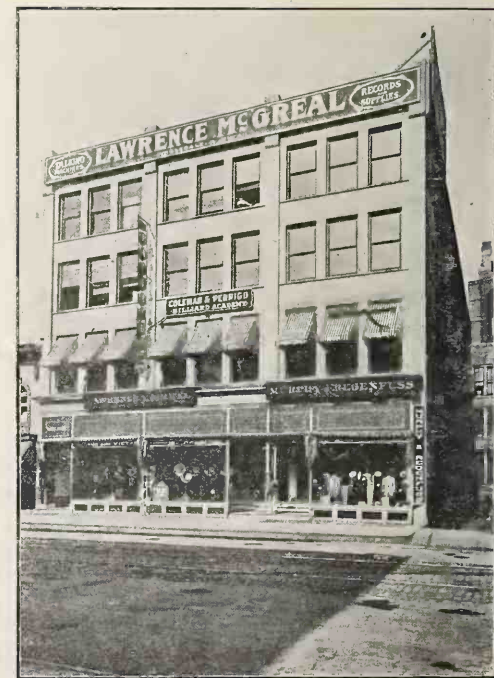
M'GREAL'S MILWAUKEE HEADQUARTERS.
