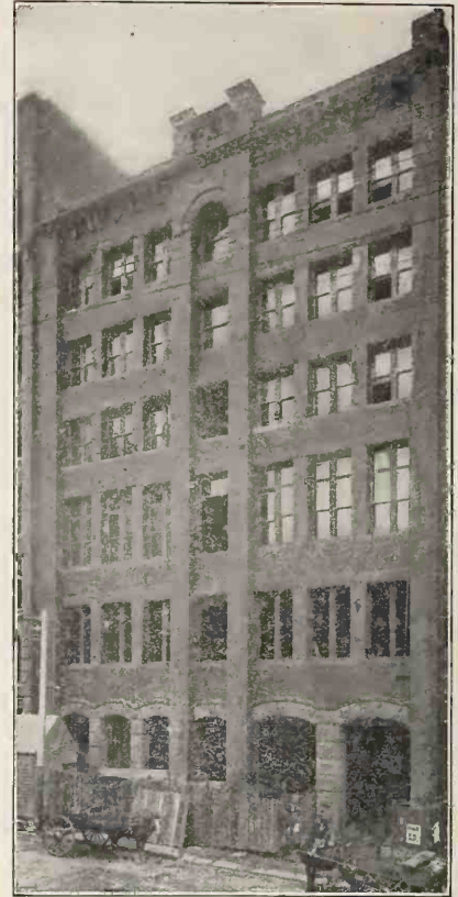
NATIONAL CO.'S AUSTRALIAN HEADQUARTERS.
