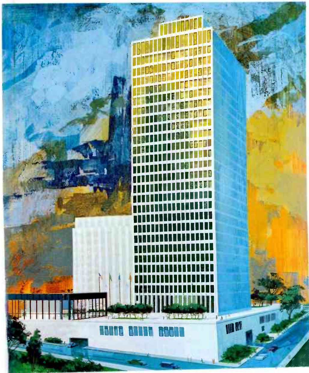
The future home of the National Life and Accident Insurance Company, now nearing completion in downtown Nashville. The building, the tallest on the Nashville skyline, will house the firm that gave WSM and the Opry birth.
