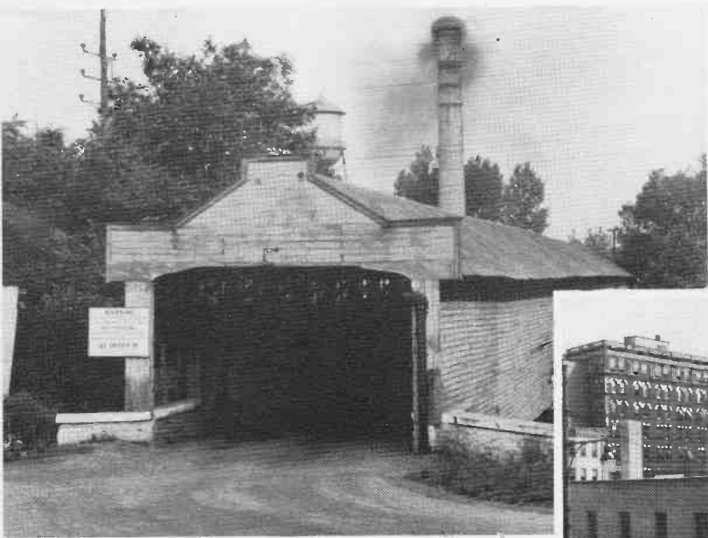
Typical of quaint old covered bridges dotting the countryside.
