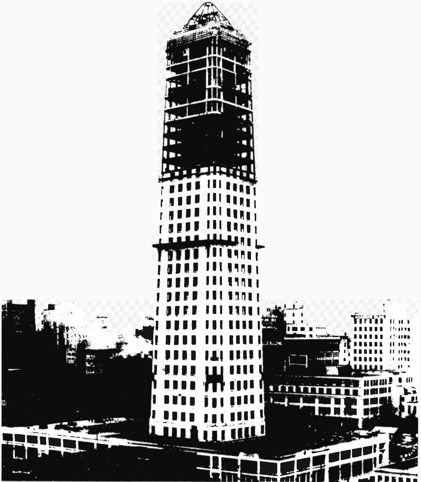
The Foshay Tower, Minneapolis, 1929, the final stage of construction.
