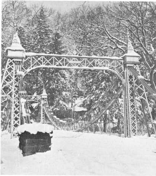
Bridge at Hiawatha Flats.
