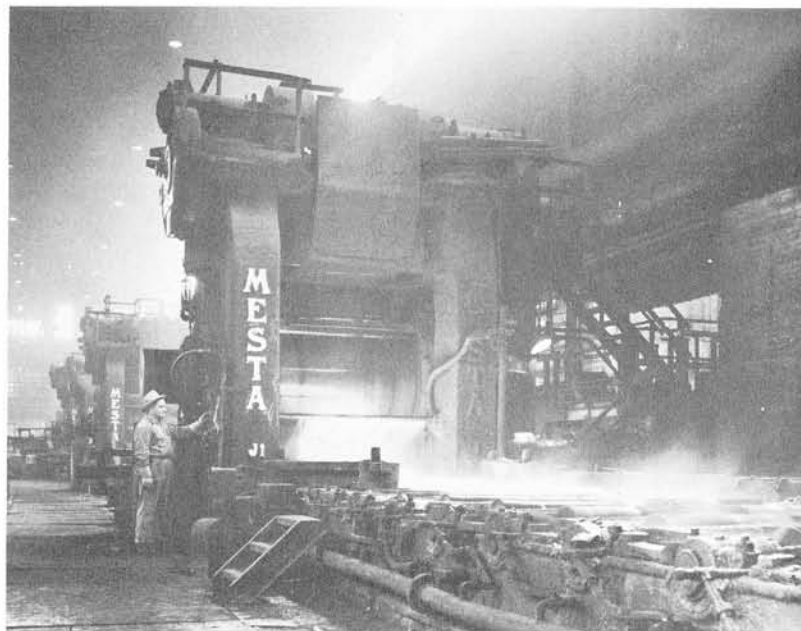
Roughing Stands of Hot Strip.
