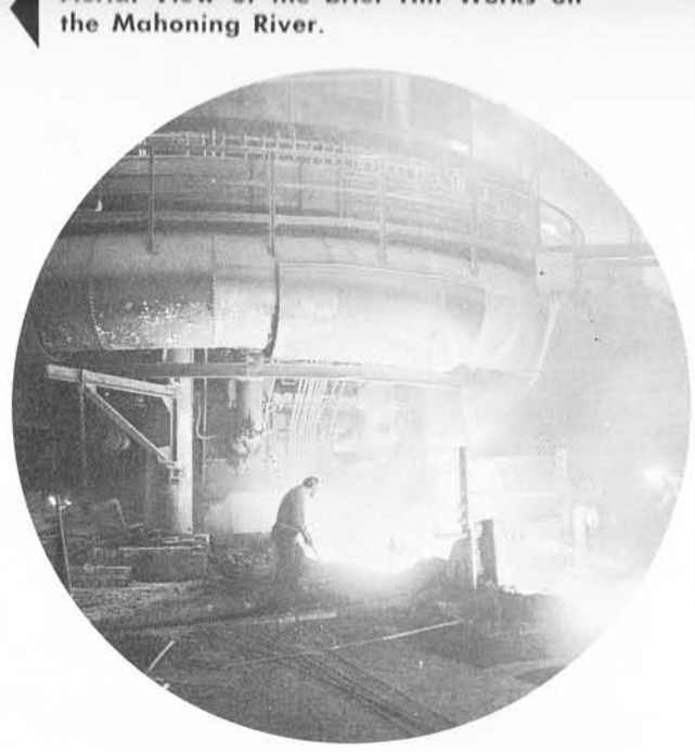
Skimming off the slag from the blast furnace.
