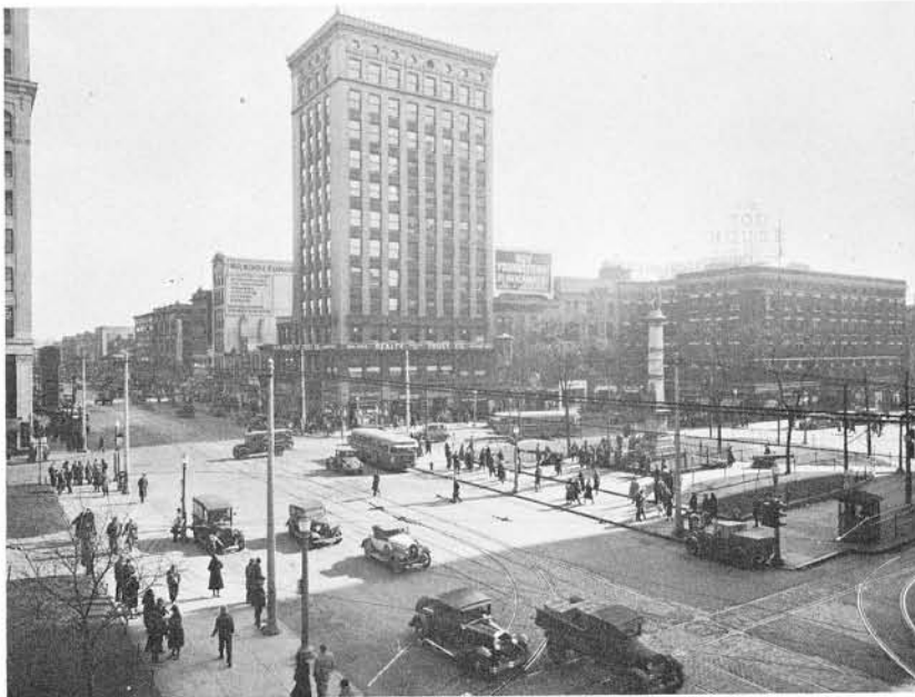
View of Federal Street with new central Bank under construction.
