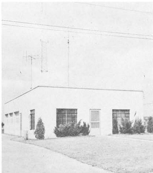
Transmitter and tower.
