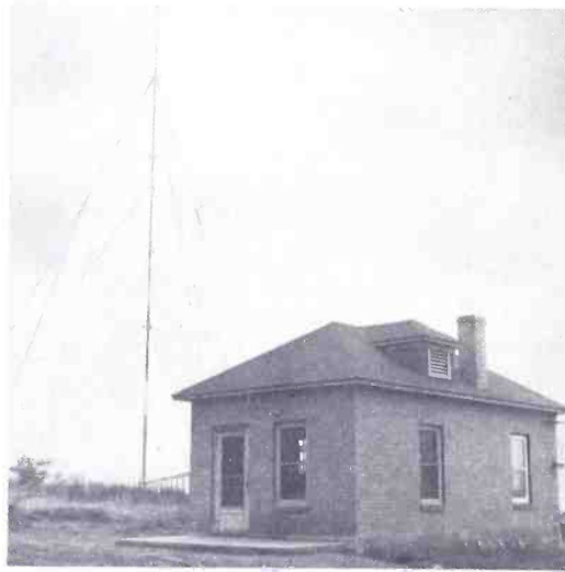
WARD's transmitter building is located on a hard-to-get at hilltop which overlooks all of Johnstown. It houses amplitude modulation transmitting equipment and frequency modulation equipment. To the left of the building is the vertical antenna for AM broadcasts.
