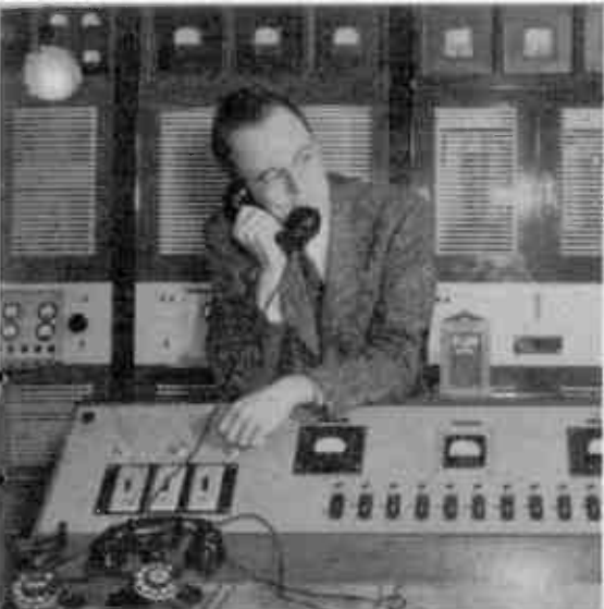
DICK FRAZIER and WIRE'S Transmitter Control panel.
