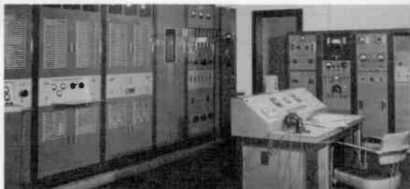
WIRE'S TRANSMITTER OPERATIONS ROOM shows the powerful 5000 watt high-fidelity transmitter at the left — and extending beyond the picture's limits. In the center is the control desk.
