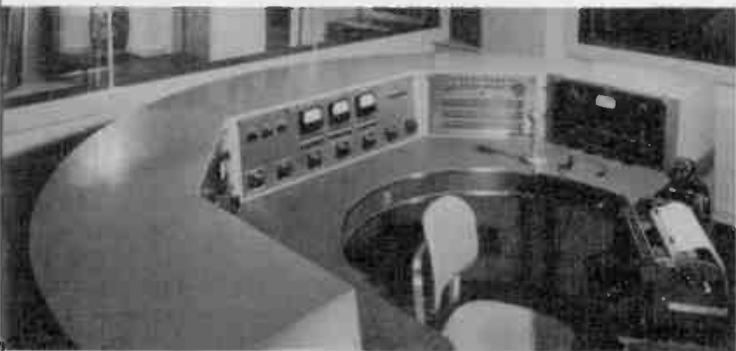
WIRE'S MASTER CONTROL ROOM at the studios atop the Claypool Hotel gives a view of each of the four modern studios. At the console shown here are controlled all local programs and those either going to or coming from the NBC Red or Mutual networks.
