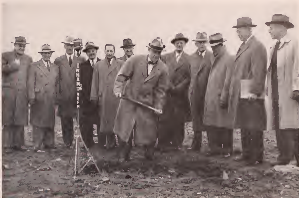
FIRST SCOOP—William Fay, Stromberg-Carlson vice-president, starts digging for the foundation of WHAM's new home. Building will also house FM and television facilities.
