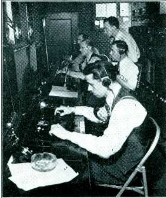
Fig. 5—The television control room. Note the two Kinescope monitors in the upper left corner.
