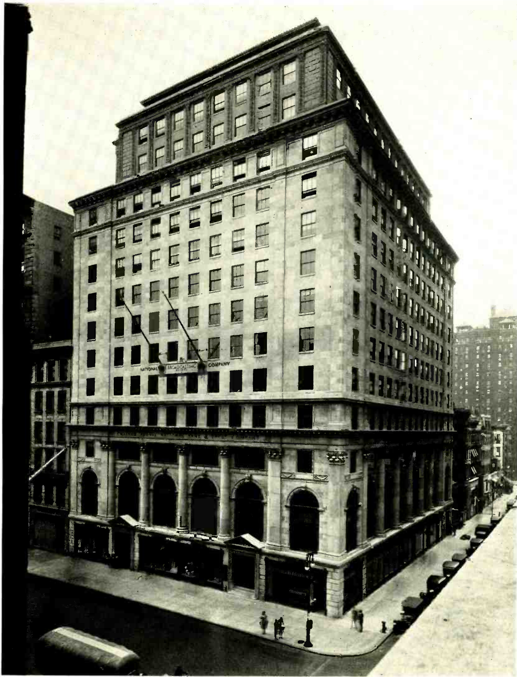
"BROADCASTING HEADQUARTERS" TODAY, THE NATIONAL BROADCASTING COMPANY BUILDING, 711 FIFTH AVENUE, NEW YORK
