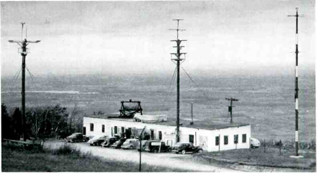
FIG. 1. FM STATION W57A IS IDEALLY LOCATED ON THE EDGE OF A STEEP CLIFF FACING THE AREA OF CONCENTRATED POPULATION. TRANSMITTING ANTENNA IS AT RIGHT
