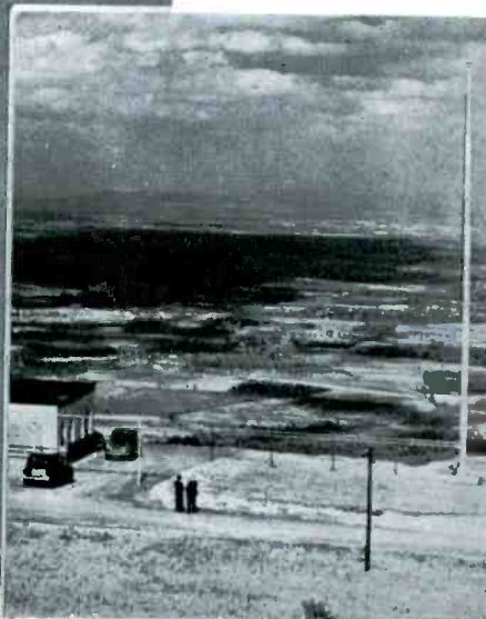
FIG. 4. CLOSE-UP OF THE ANTENNA USED AT THE HELDERBERG STATION FOR TESTING THE 50-KW. TRANSMITTER, AND A VIEW FROM THE STATION OF THE VALLEY BELOW
