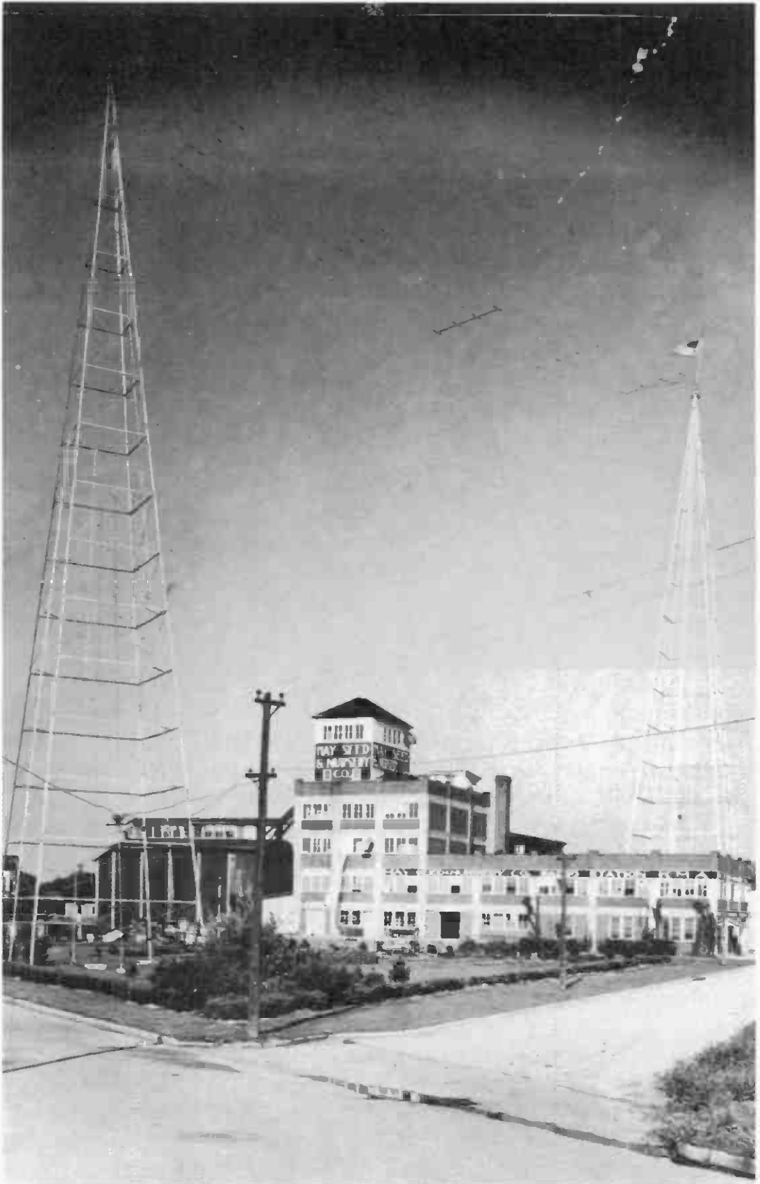
One of the original towers of radio station KMA rose above the roof of the seedhouse, while the other stood west of the building. Four wires suspended between the towers completed the array.
