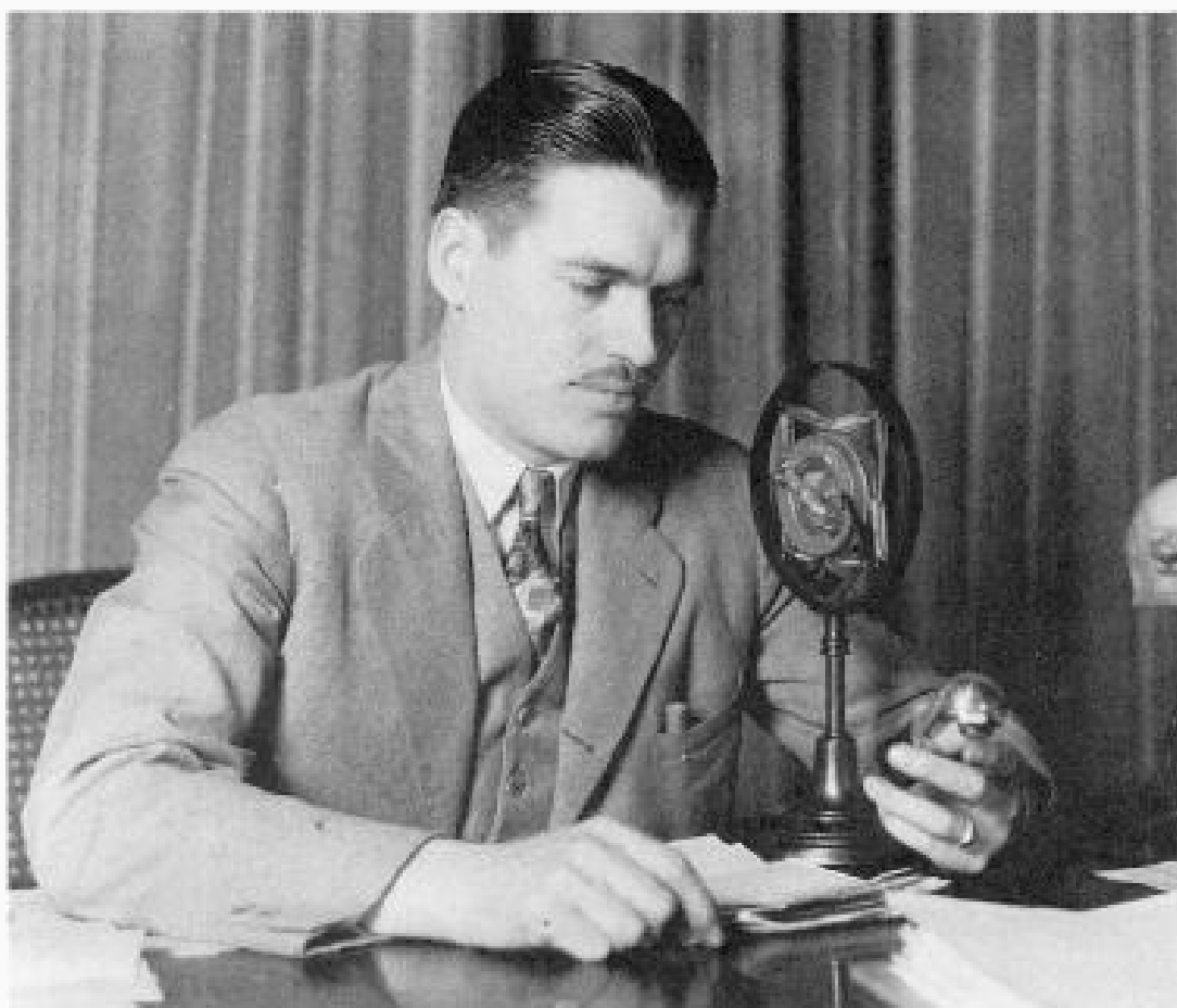
As KMA's first engineer, J. C. "Cy" Rapp directed the installation of the original transmitter.
