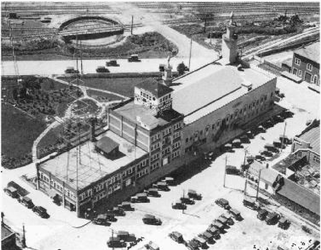
The May Seed & Nursery Company complex in late 1927 included the seedhouse and, sporting a Moorish minaret, the new Mayfair Auditorium. The rumble of trains on the tracks west of the building sounded in the microphones on the Mayfair stage.
