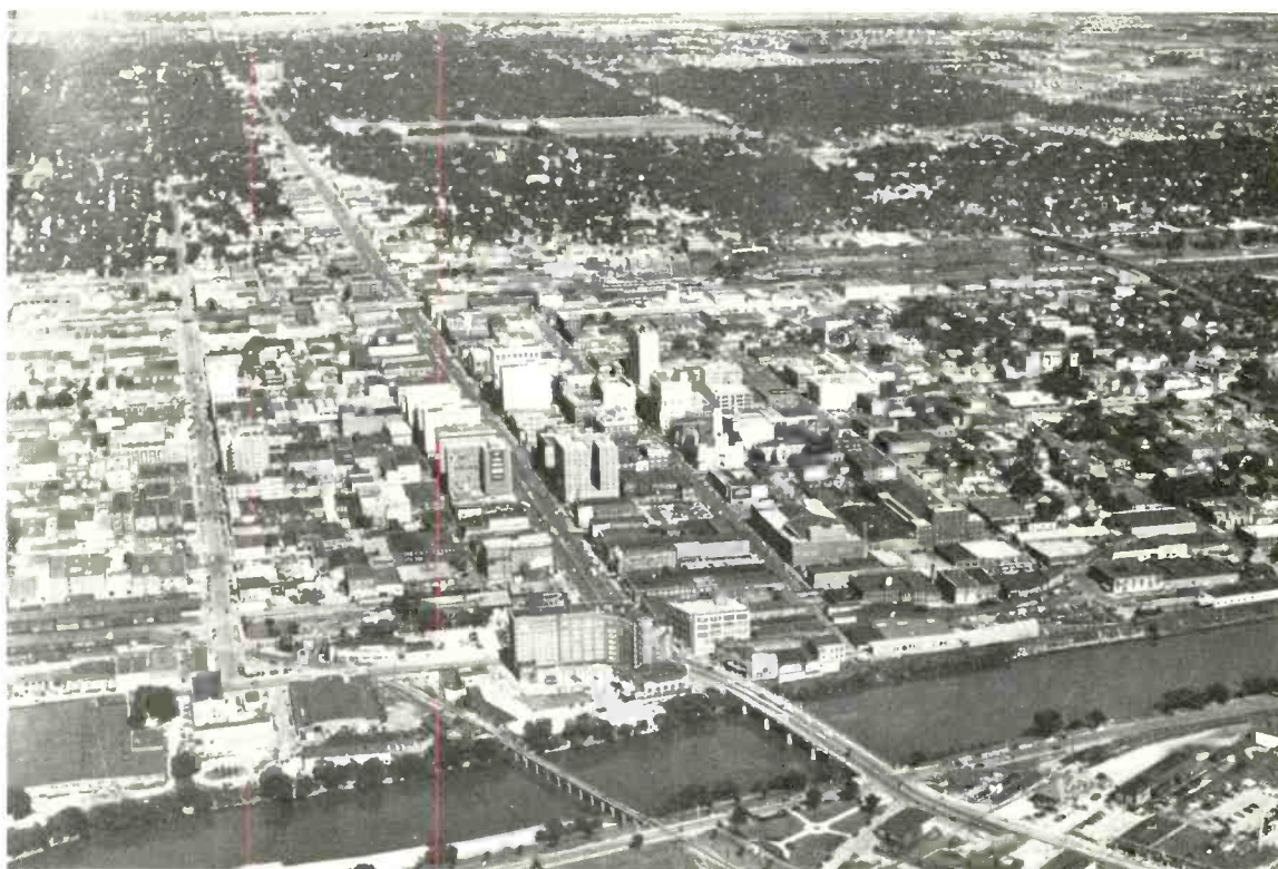
An airview of Wichita's downtown and suburban area. In the foreground is the Arkansas River flanked by some of the industrial companies. The city is divided by Douglas Avenue. Hundreds of stately trees that help to make Wichita one of the most beautiful cities in the country are visible in the background.
