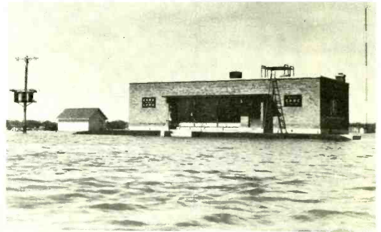
Transmitter equipment was seriously threatened and partially damaged by the raging Red River during Manitoba's flood of 1950. The high water mark can be seen on the building as the flood water recedes.
