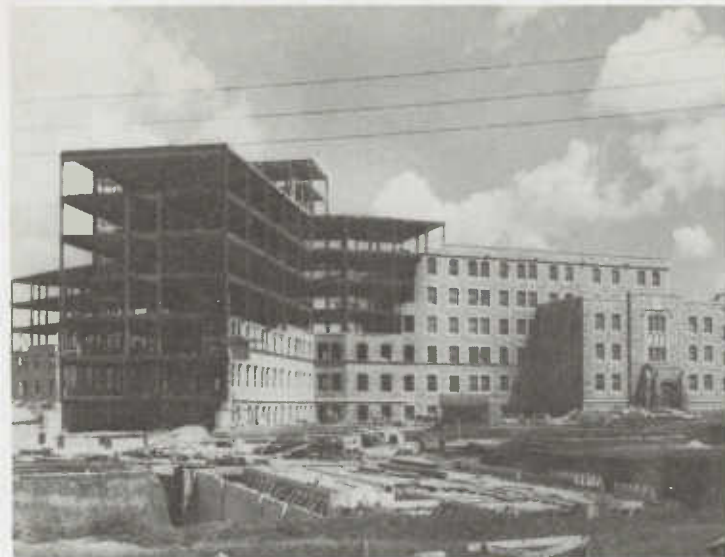
University Hospital under construction
