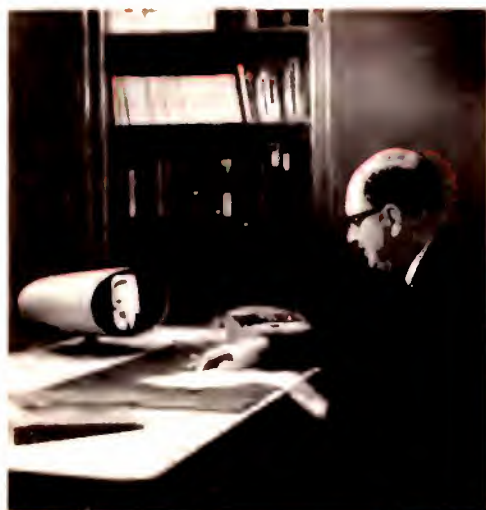
L. H. Meacham at his desk in Bell Telephone Laboratories, Holmdel, N.J., talks with and views A. D. Hall on the experimental Picturephone. Both engineers helped develop the visual telephone system. Meacham is using hands-free Speakerphone service, while Hall at Murray Hill laboratories uses the handset.
