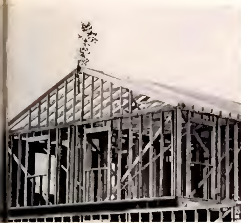
The walls begin to rise and soon the roof tree's overhead
