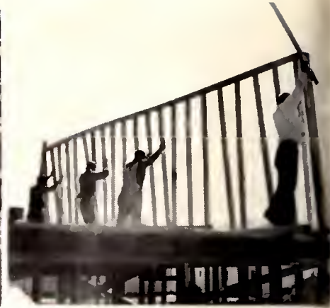
As all the builders' men start working hand-in-hand
