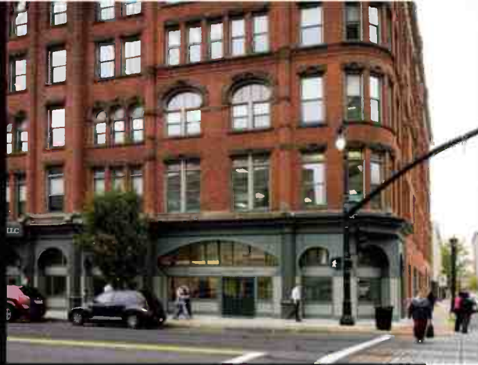
New England Public Radio's beautiful new facilities in a historic Springfield, MA building presented some interesting challenges.
