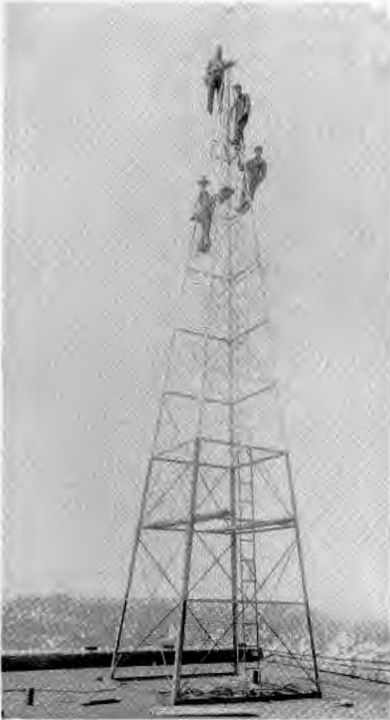
One of the two fifty foot windmill towers supporting WBTM's 'T' type antenna back in the thirties. This was a far cry from WBTM's three tower directional array of antennas as used today.
