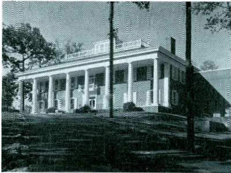
A strikingly different structure that could easily pass as a mansion for Scarlett O'Hara, was formally opened in Atlanta by WSB on Sunday. Designed and built by the Austin Company to harmonize with Atlanta's traditional southern charm, the authentically Georgian structure has an estate-like setting on an historic hilltop.
