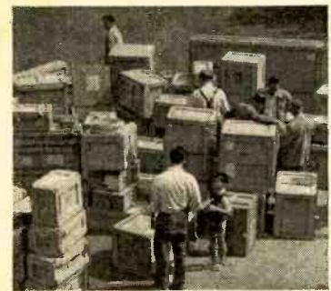
Part of the 401 cases of RCA equipment shipped to Berlin for television demonstrations.
