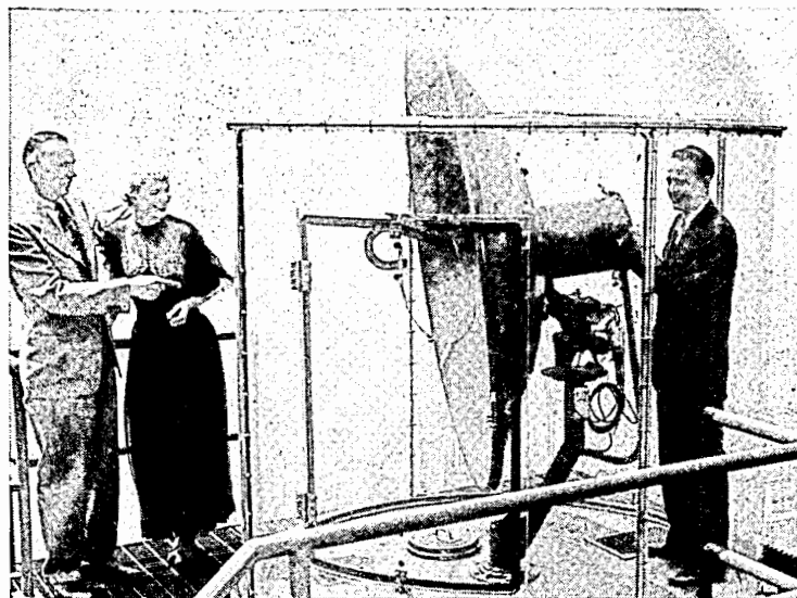
Chester Rackey and Kyle MacDonnell, NBC-TV, watch a demonstration by Robert H. Barnaby, NBC engineer, of relay equipment installed in one of two radomes atop the RCA Bldg., N. Y. Equipment enables web to receive video programs from temporary field locations within a 30-mile radius.
