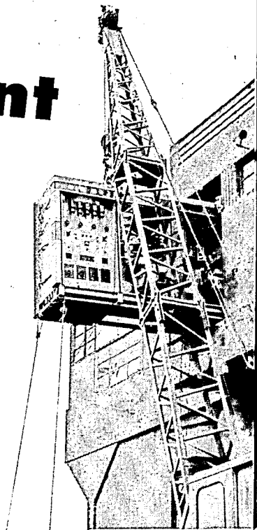
EASY DOES IT! This shot shows one of the units of the new KGW transmitter being derricked through a second story window of the transmitter house. The new installation will give KGW the most efficient transmitting equipment yet developed by the radio industry.
