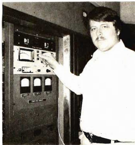
Checking the antenna monitor of KEX's 1947 Westinghouse 50-HG-1 transmitter is author Donn Werrbach.
