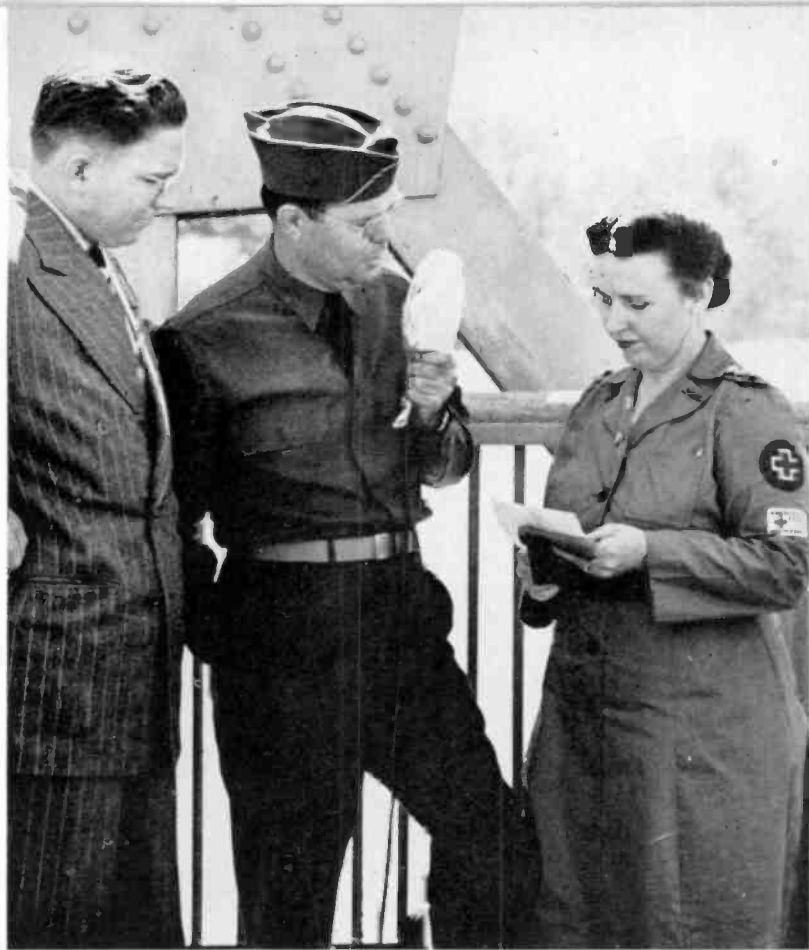
FLOOD WRECKS station tower but information and directions to public continue through mobile transmitter.
