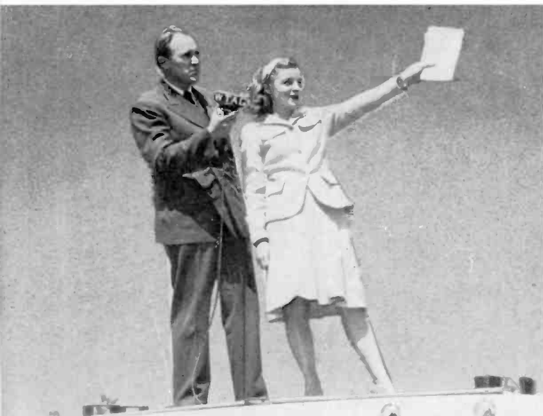
FIRST DYNAMITE BLAST in construction of city's first airport described with "remote" equipment.
