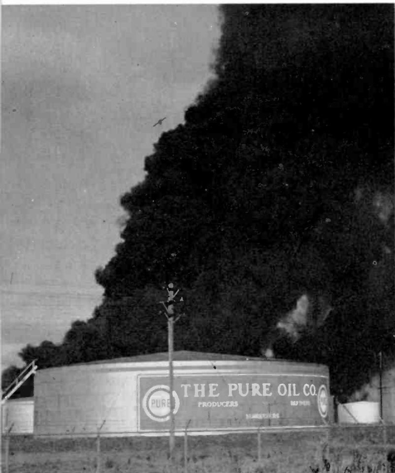
100,000 BARREL oil tank fire sends large column of smoke over alarmed southwestern community.
