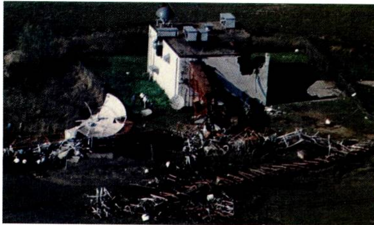
Upgrading the tower of KNOE-TV led to the death of a crew member
