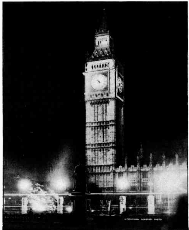
Big Ben, the chimes from which close the programs broadcast from England, is one of the historical landmarks of London. Built in 1858, it is still reputed to be the most powerful striking clock in the world. The bell weighs 13½ tons, the hammer 400 pounds. Its hour hand measures 9 feet long, and its minute hand 14 feet.
