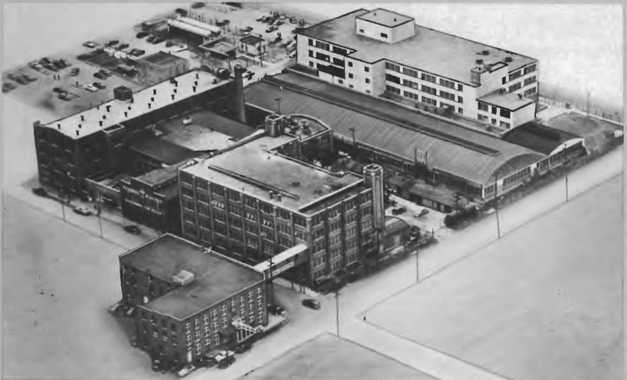
To meet requirements of the Armed Services for high-reliability tubes, General Electric enlarged its factories such as this one in Owensboro, Kentucky. By the middle of 1952, production of G-E Five-Star tubes was increased 5 to 1 over 1951.
