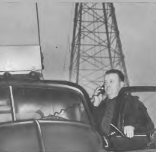
Remote Control—Unattended Stations
