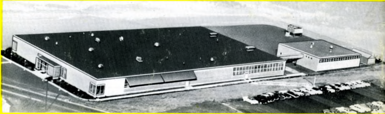
SEMICONDUCTOR MANUFACTURING FACILITY, SLATERSVILLE, RHODE ISLAND
