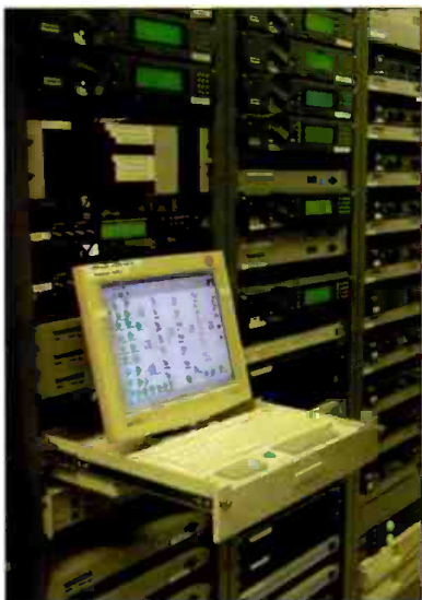
The Tandberg System Manager at WKCF Orlando includes encoders with internal remultiplexers for each remote site.
