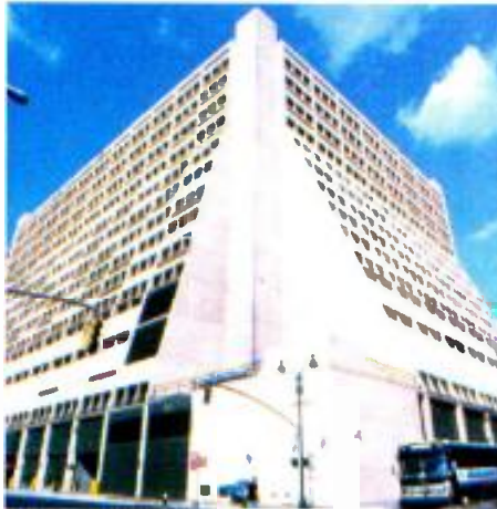
WNET's new state-of-the-art facility will feature a Sony-equipped HDTV cutting room and Tektronix master-control gear.
