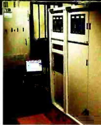
WSB-TV will begin moving into a $35 million all-digital facility in May. At right is the station's new DTV Harris 100 kw transmitter, outfitted with an ATSC-compliant encoder.
