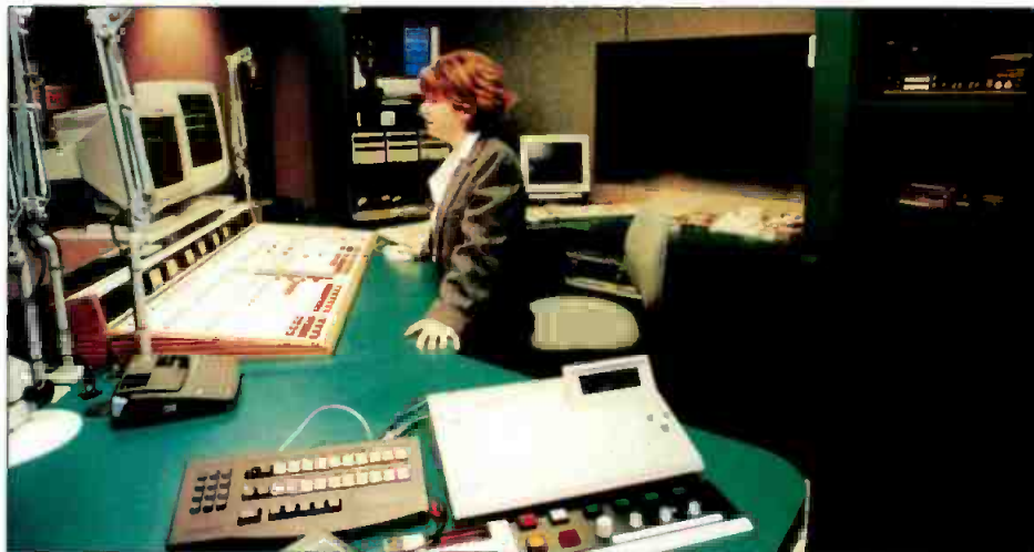
EZ Communications' renovations to KMPS AM-FM Seattle's on-air studio bring new digital console equipment and computerized scheduling capability to the stations.
