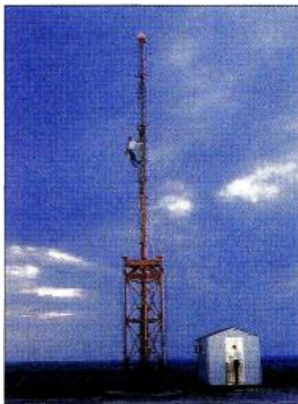
Broadcasters hope co-locating adjacent channel HDTV and NTSC antennas on a single tower will combat interference.
