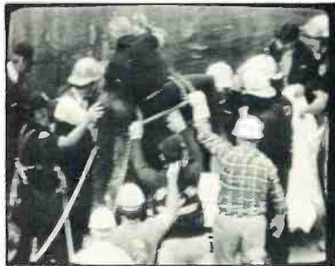
WKYC-TV at a construction site explosion
