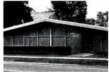
New home. Corporate headquarters of Lima Broadcasting, licensee of WIMA-AM-FM Lima, Ohio, has expanded to occupy this $225,000 facility at 667 West Market Street, Lima. Building was designed by Bowman and Armstrong; architects. Installation of MW-1 Gates transmitter is expected this month.
